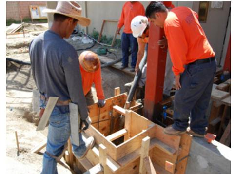
*Pumping concrete into the elevator structure footing.*
